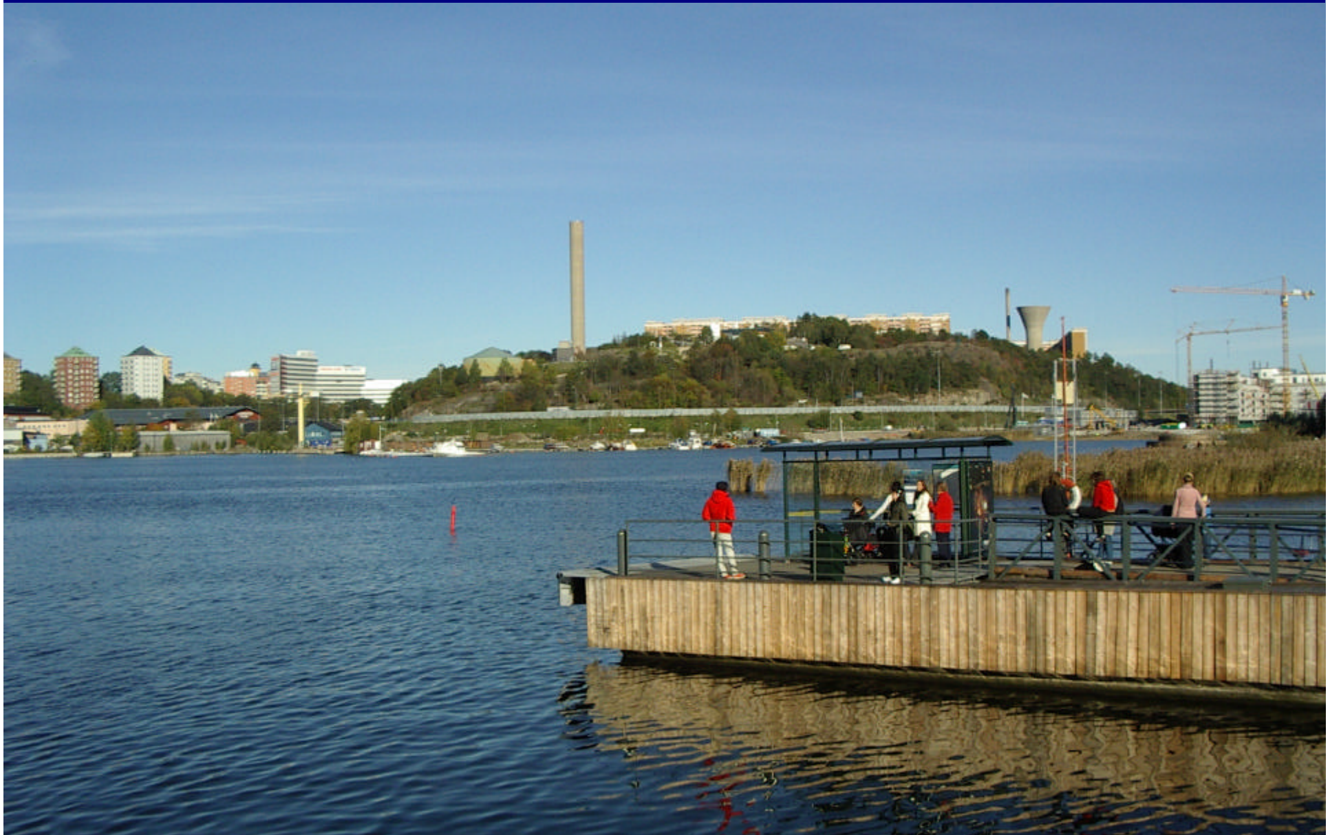
Stockholm's Henriksdals treatment plant
