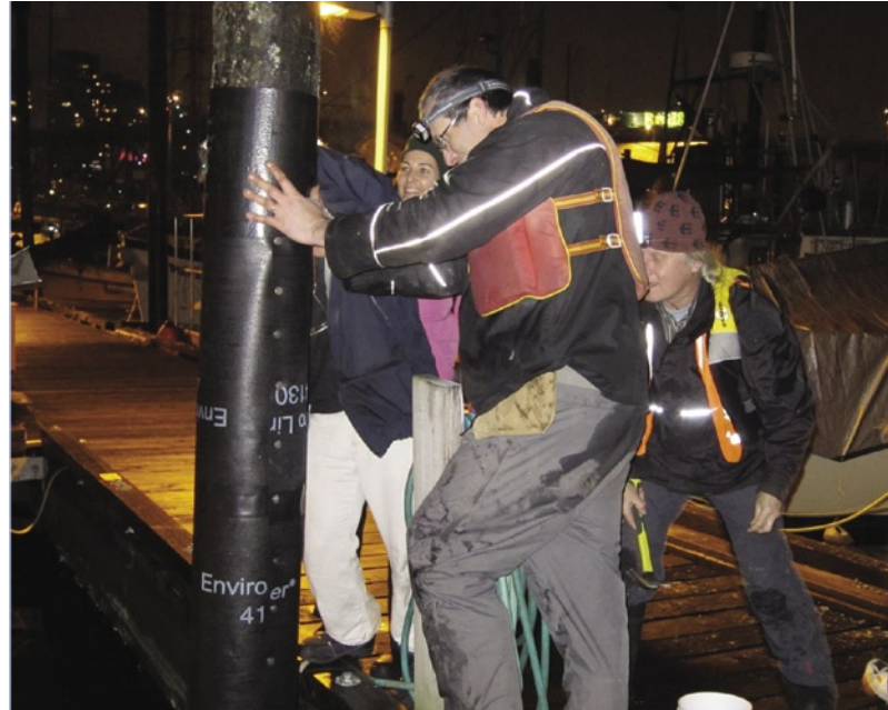
Fisherman's Wharf in False Creek coated creosote pilings with a protective liner which boosted the herring egg hatch rate.
