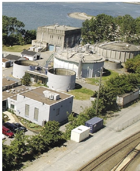
The existing Lions Gate sewage plant.
