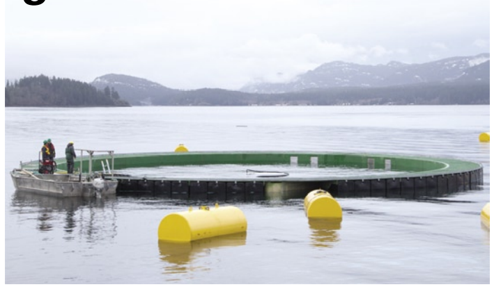
Closed containment tank at Middle Bay, near Campbell River.
