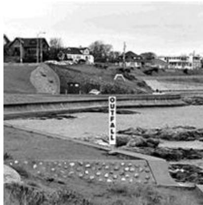
CREDIT: Ray Smith, Times Colonist B.C. Environment Minister Barry Penner has expressed concern about contamination around the Clover Point sewage outfall.
