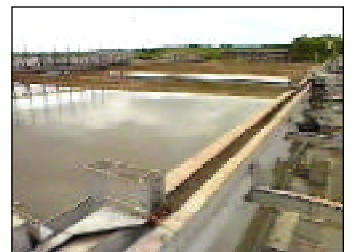
Primary treatment: solids are separated from liquids in a settling tank.
