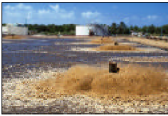
Air-activated sludge lowers the dissolved oxygen content and faecal coliform levels.
