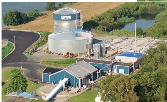
Kristianstad Sewage/Biogas Plant
