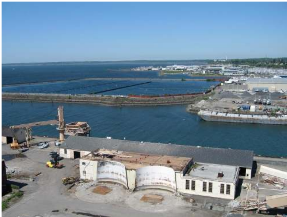
Whatcom Waterway in Bellingham Bay (Port of Bellingham)
