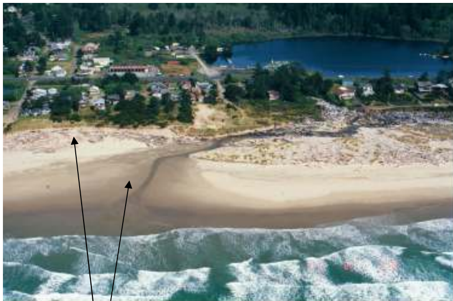
Shoreline and dune erosion
